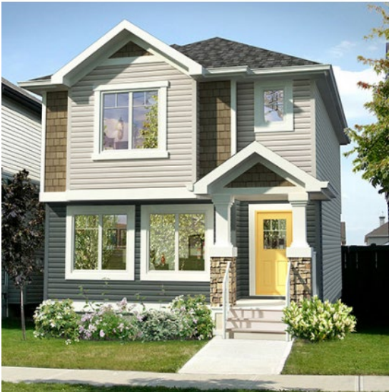
Pictures are general examples only. All Guidelines must be strictly adhered to and may not be reflected in the elevation examples
